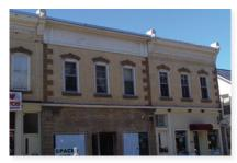
as well as the date block of 1883 on the centre building. The differences in the upper cornices indicate that the building was built in two or three phases.
